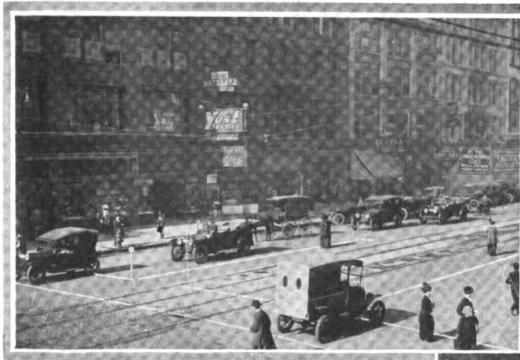
Pedestrian safety lane and street car safety zone on Woodward avenue and Grand River
